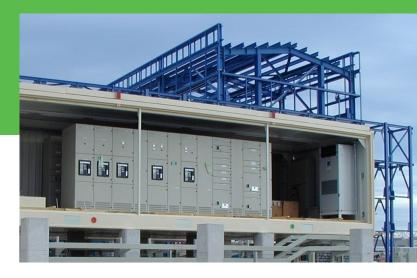
With the installation of complete electrical systems into POWER HOUSES, FEAG offers a variety of factory-tested solutions in a ready-to-operate system including air conditioning and the suitable housing - complete & prepared for the connection of field cables at site. The installation effort for the user is significantly reduced, the assembly time is shortened and the planning and scheduling risk is minimised.
